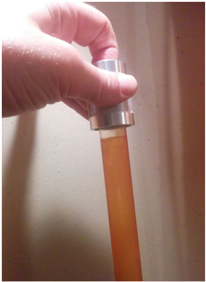
Make sure that the ultraviolet light bulb sleeve is cleaned on a regular basis. If the sleeve becomes dirty, the UV light cannot properly inactivate germs, allowing contaminated water to flow through untreated.
