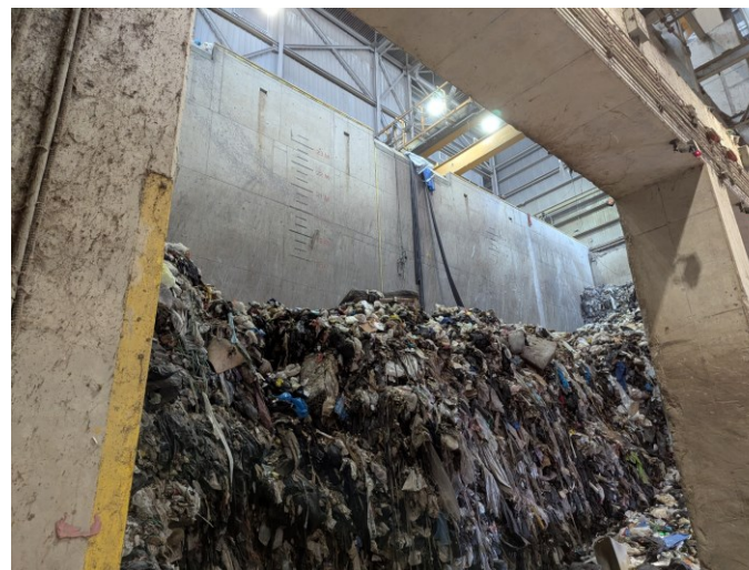
Photo 36: View of waste bunker within Tipping Building.
