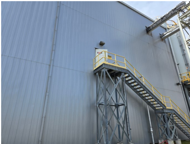
Photo 23: View of open Residue Building Door.
