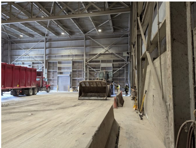
Photo 39: View of loader in the Tipping Building.
