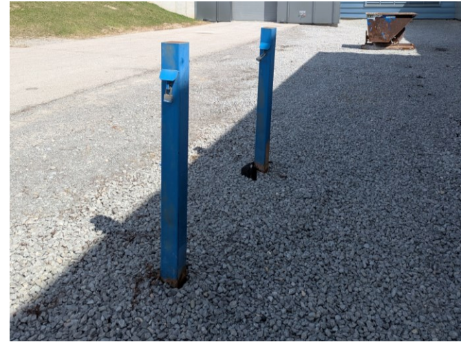
Photo 38: View of monitoring wells in good condition near the Diesel Generator.
