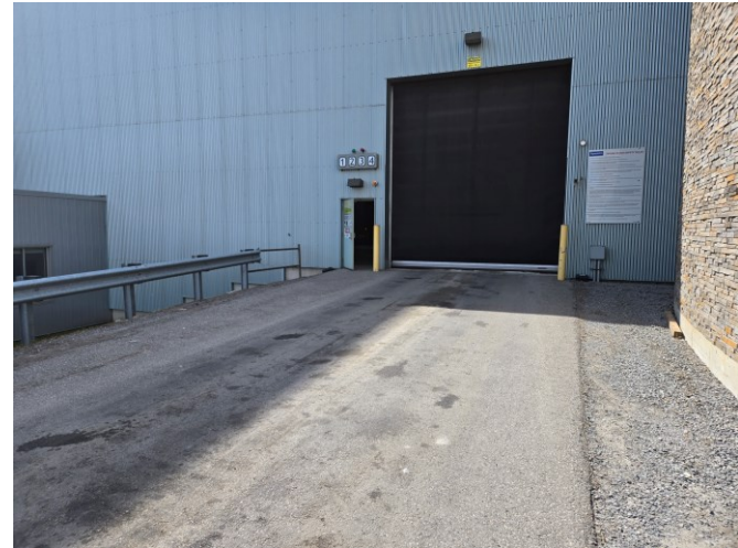
Photo 14: View of repaired Tipping Building vehicle door and ajar person door.
