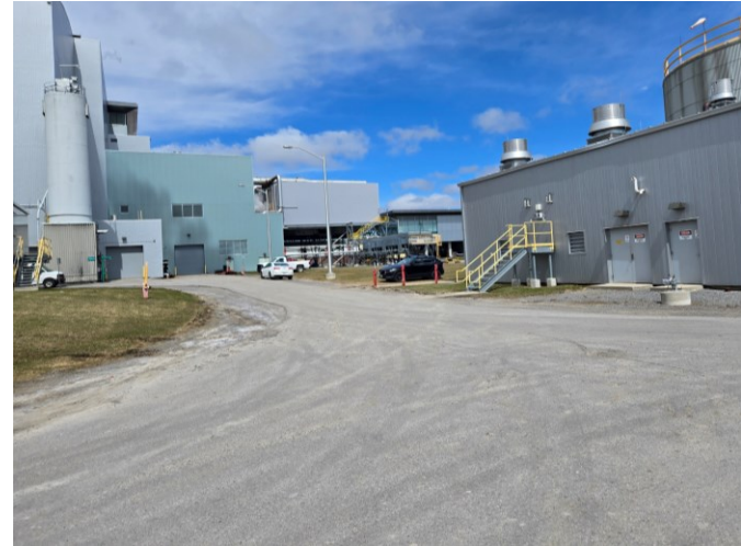
Photo 22: View of contractor vehicles parked on grass near the Fire Pump House.
