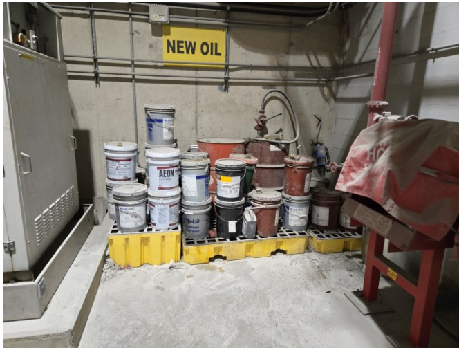
Photo 17: View of the new oil storage area.
