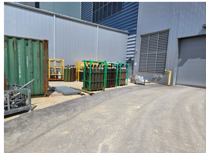
Photo 12: View of un racked compressed gas cylinders south of the Grizzly Building.
