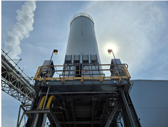
Photo 13: View of open Pozzolan silo door.
