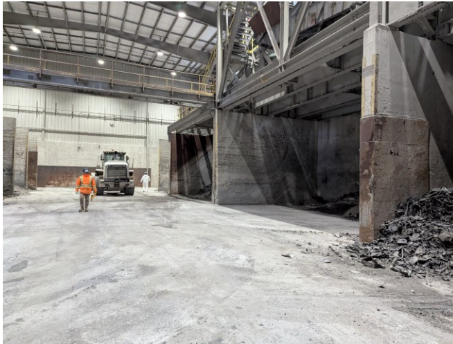
Photo 37: View of loader in the Residue Building.
