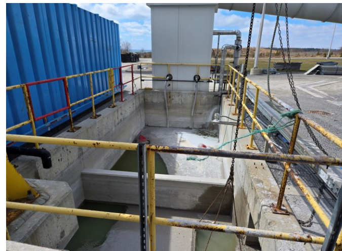
Photo 34: View of the wastewater settling basin.
