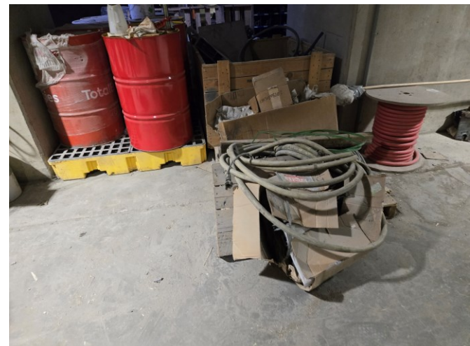
Photo 32: View of hoses in the Boiler Building.
